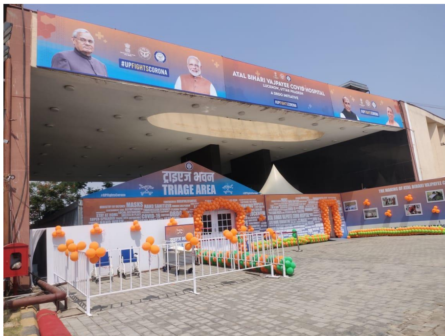
Photo 5.2: Main Entrance of Atal Bihari Vajpayee COVID Care Hospital, Lucknow, Uttarpradesh
